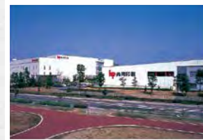
Panoramic view of Goka Plant
