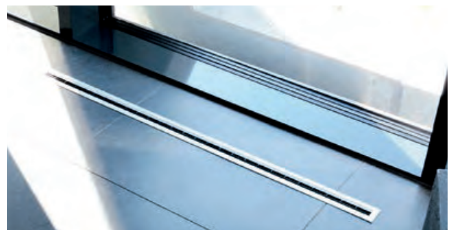
The ventilation unit Evotherm 1000 F – shown here – and the heat exchanger were both installed flatly on the ceiling of the technical facilities room to save space. From here, the air is pumped into the individual rooms where only discreet slits in the floor indicate the presence of a controlled ventilation system.
